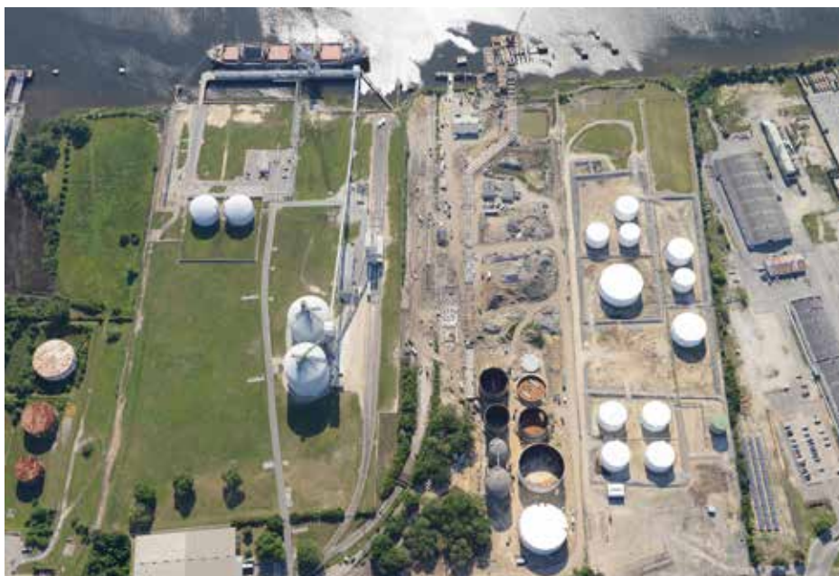
Status on progress mid-May 2013
