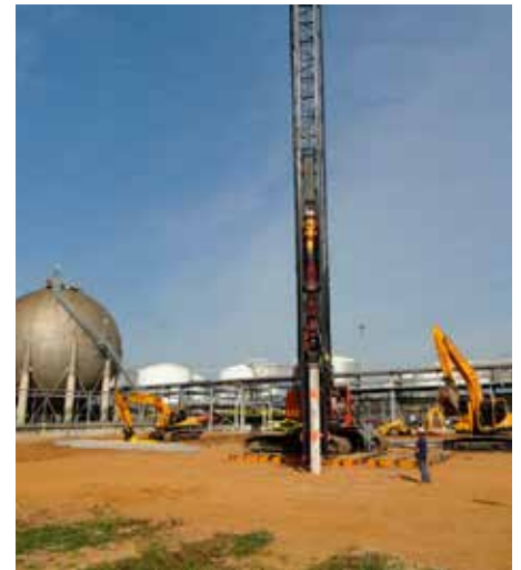
First 15.4 meters (50 foot) piling for Bay 10
