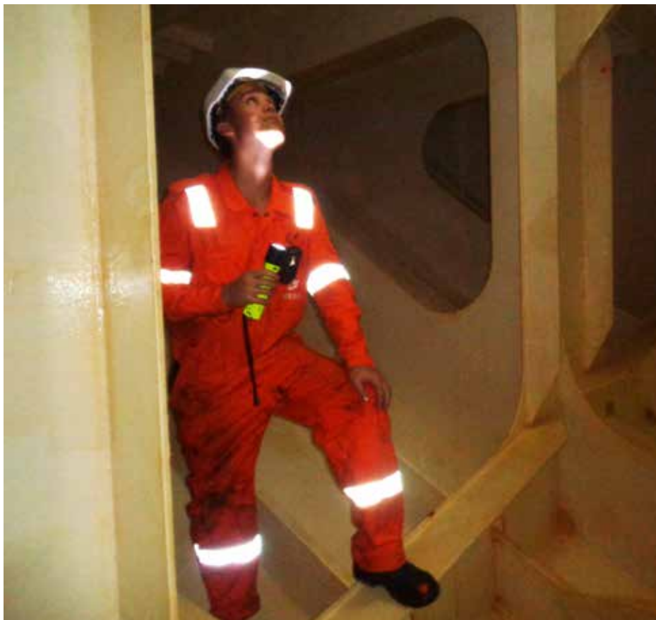
Ole Magnus is inspecting one of the watertanks on board Bow Flora
