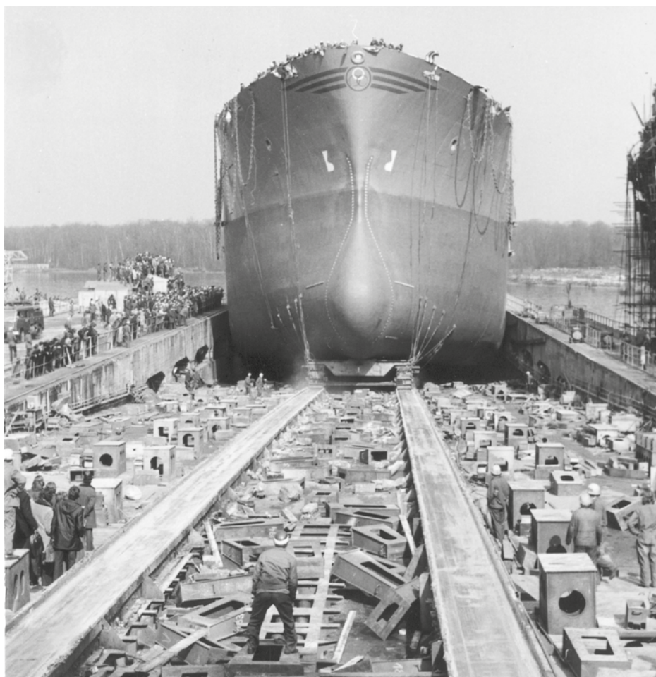
Launching one of the B76-skip. The Polish shipyard delivers all 12 ships within the span of a very hectic 26-month period, from November 1975 – on average one ship every 75 days
